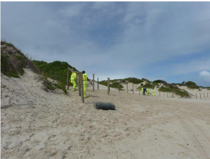
The path 16 blowouts are at the closest point between the ocean and West Coast Highway. We plan to lay about 1600 m<sup>2</sup> of coir matting behind fences up the dunes and then plant the strips of matting with tough plants like spinifex to arrest the blowouts and revegetate the dunes. It will take many years for the vegetation to grow back to do the job, but we need to start the process. The blowouts are exacerbated by fitness enthusiasts running up the dunes and other beach users so
